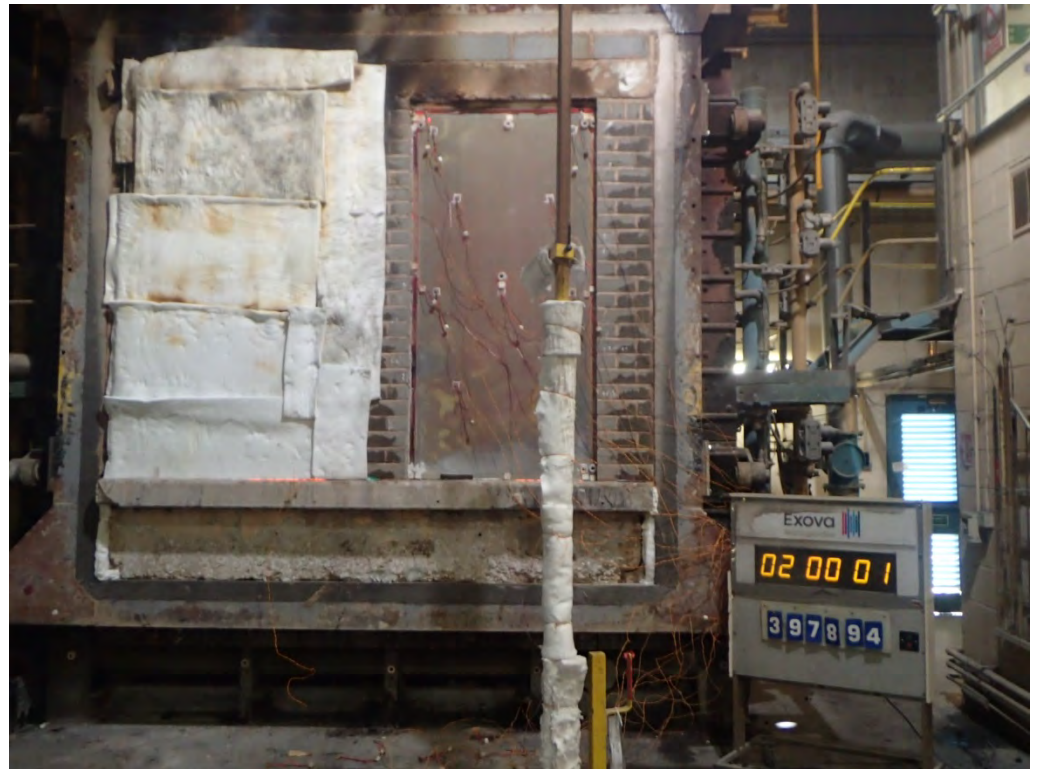
The unexposed face of Doorset B after a test duration of 120 minutes
