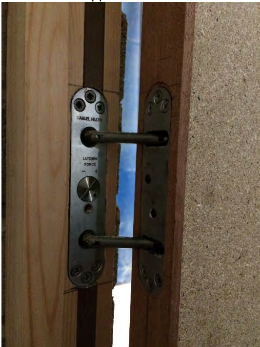
Concealed closer installed – Doorset A
