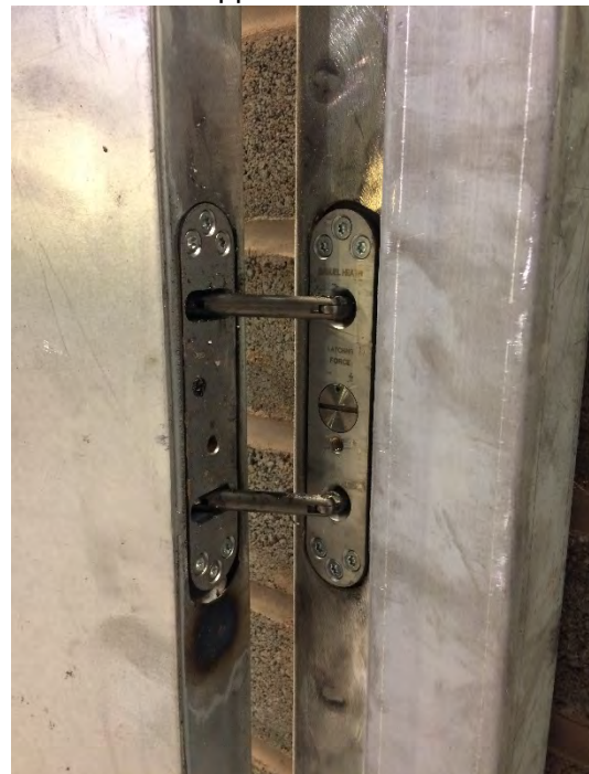
Concealed closer installed – Doorset B
